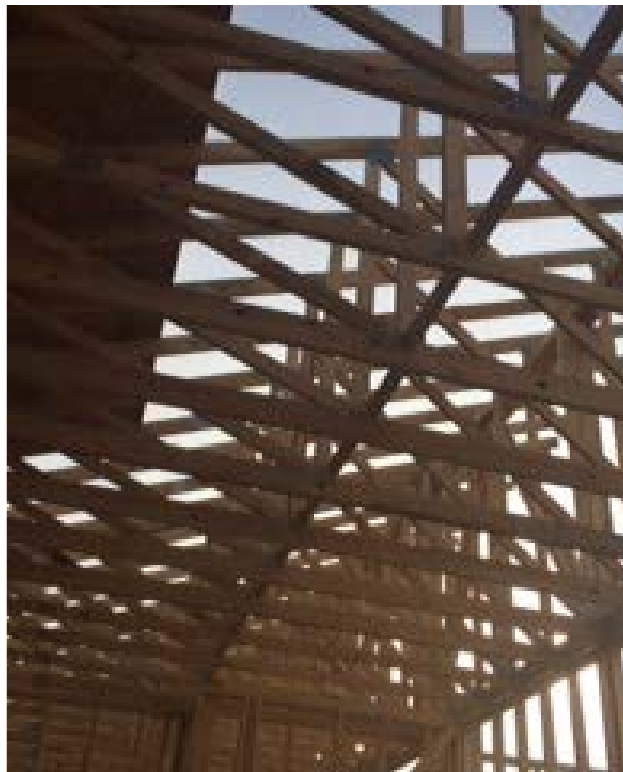
Almost ready to deck before adding the roof.
